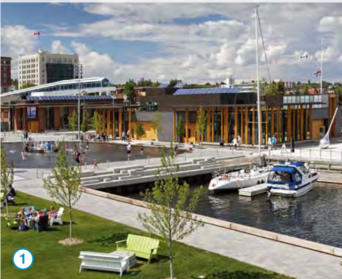
New Marina building with Seniors Centre
