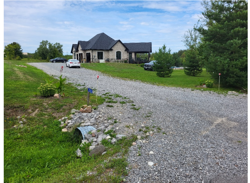
Existing dwelling and driveway
