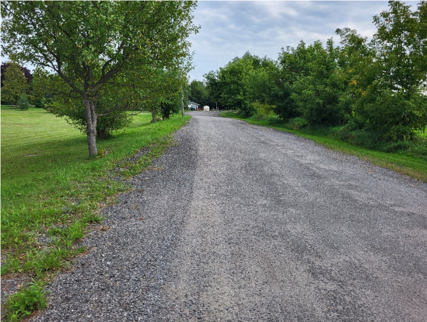
Mueller Lane, south view
