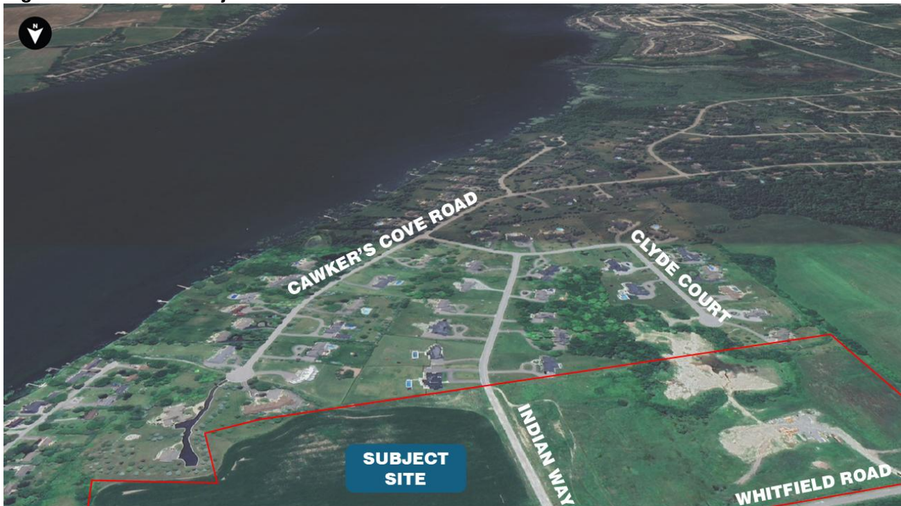
Figure 4 – South of Subject Site
